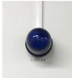
In rooms where liquid nitrogen is handled there is an alarm that is activated if the oxygen level in the room drops too low.
