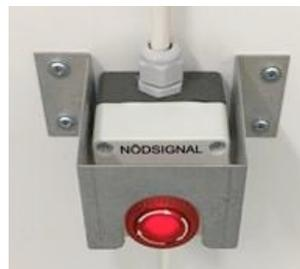
In freezer rooms there are security alarms with red push buttons. Alarms are indicated locally by sound and a red flashing light outside the room. The alarm signal is forwarded to the Biomedicum security guards. Alarms are reset inside each room by pressing the green reset button
