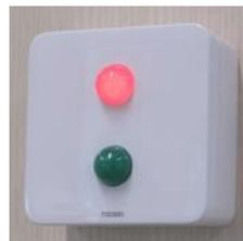
Cell culture labs and isotope labs are equipped with a pressure deviation alarm. The pressure deviation alarm is local and is indicated
